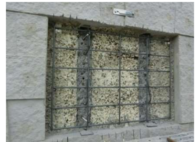
(c) 鉄筋の配筋
